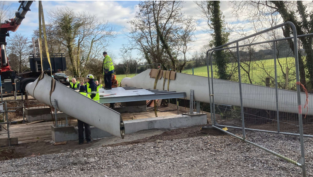
Blade Bridge Middleton-Youghal Greenway
